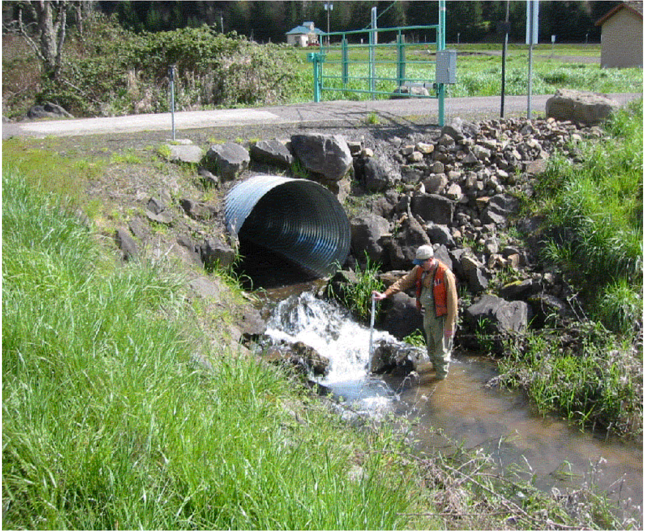
FIGURE 4. U.S. BUREAU OF RECLAMATION ROAD CROSSING AT THE END OF THE REACH 1 CREATING A POTENTIAL BARRIER TO FISH PASSAGE AT LOW FLOWS.
